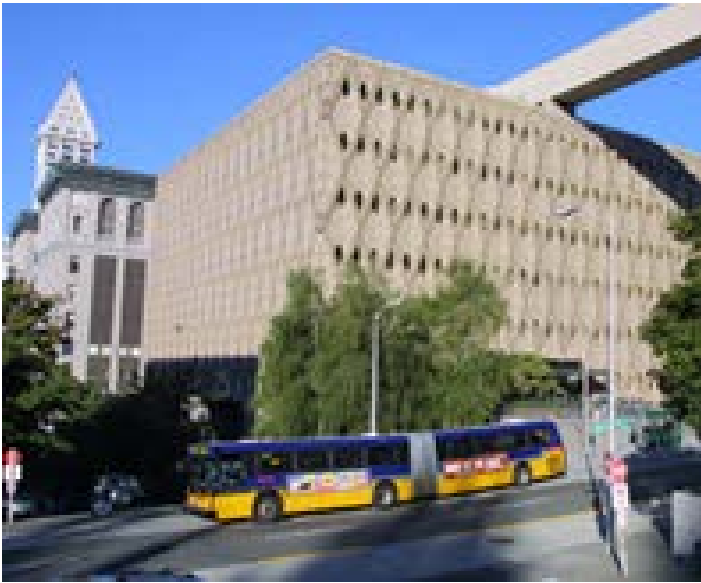
The new system took into account not only County administrative buildings but also fleet management facilities.
