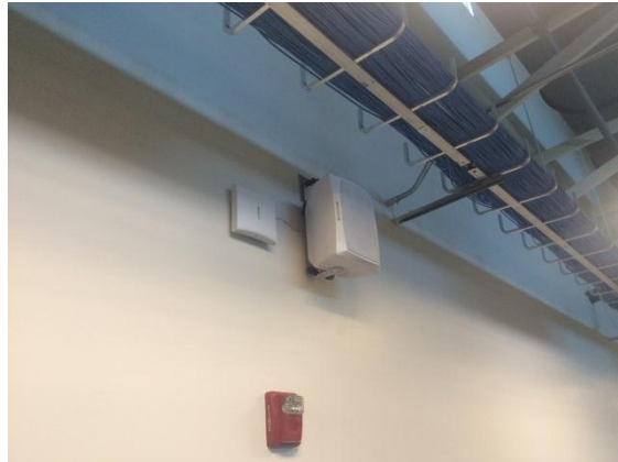
PG9920 Installed on 2 nd Floor.
